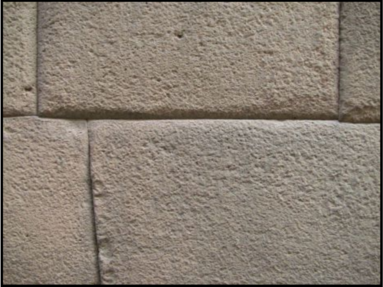
Wall detail at the Coricancha in Cusco Peru
