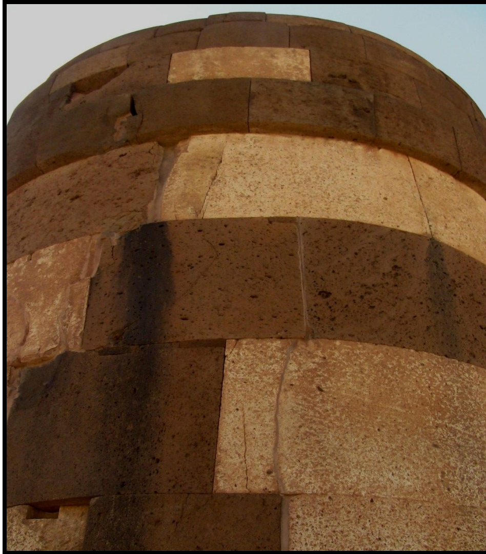
Tight and mortar free basalt stones of Sillustani
