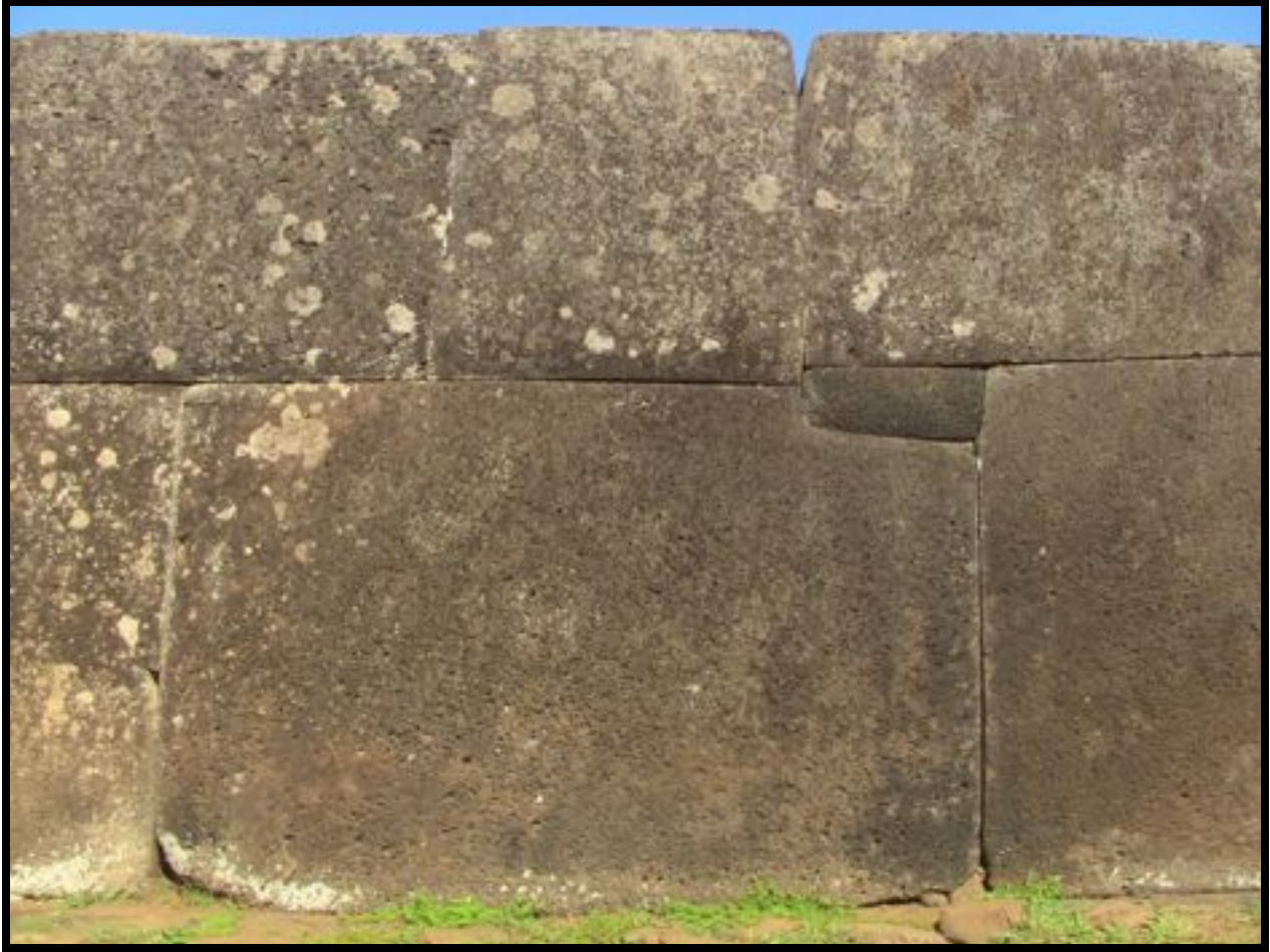
The very tight fitting basalt stones of Vinapu
