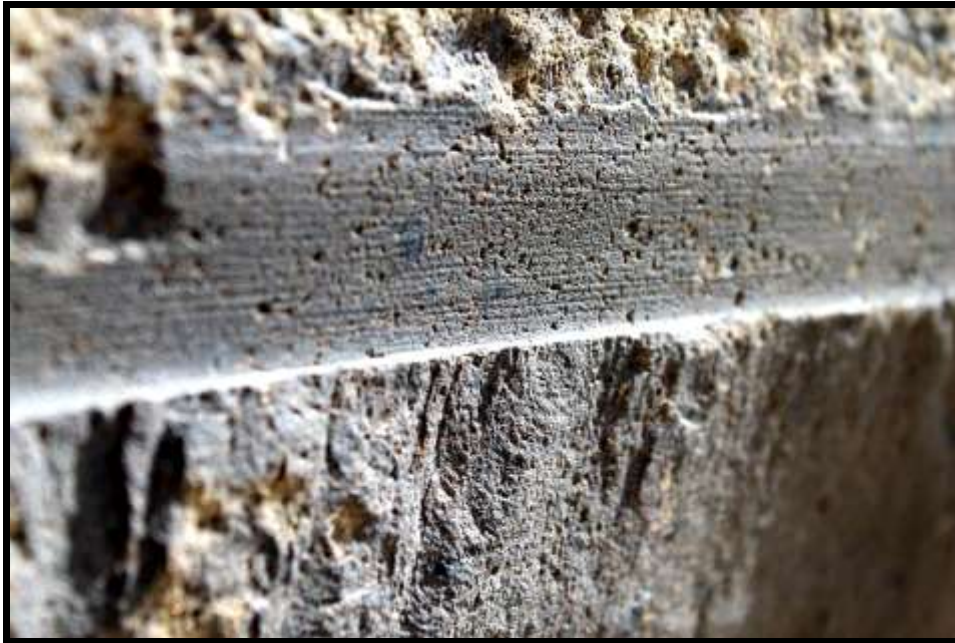
Detail view of the path of the saw
