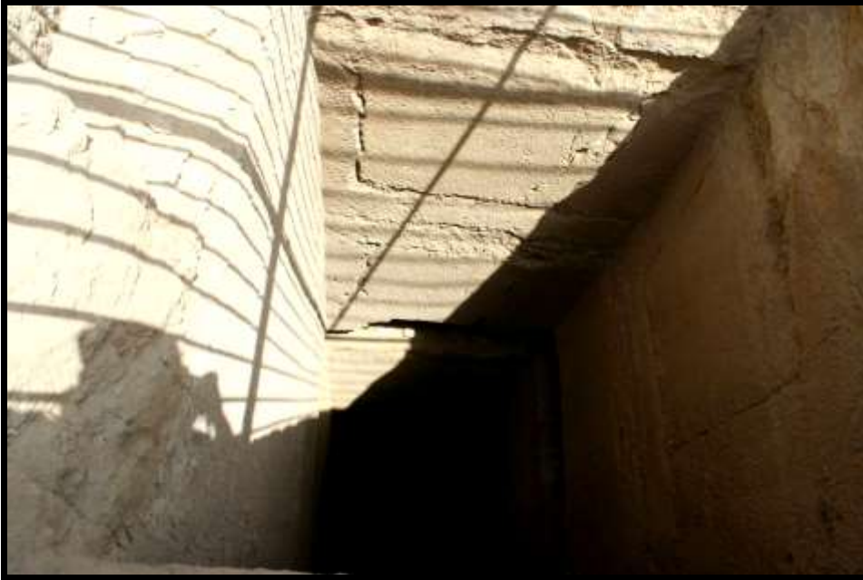
View looking down into one of the shafts
