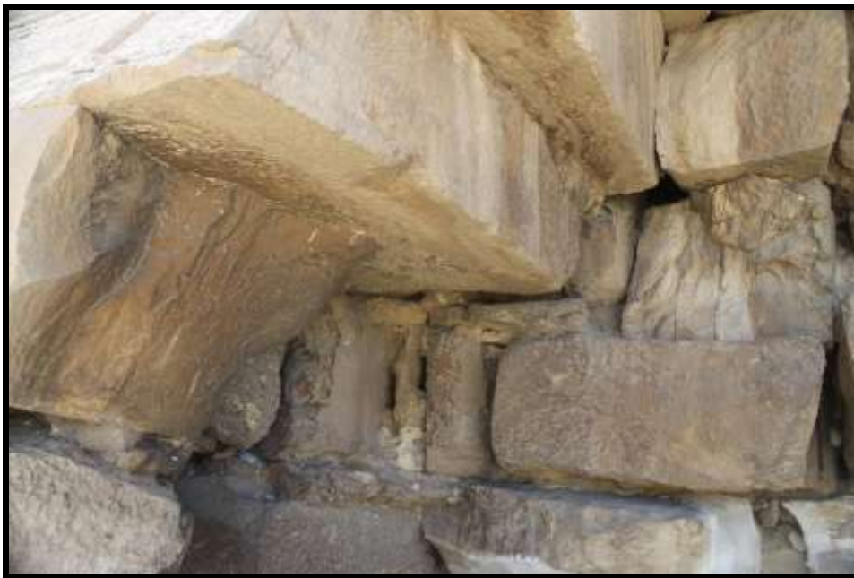
Inner stones of the Bent Pyramid with traces of concrete
