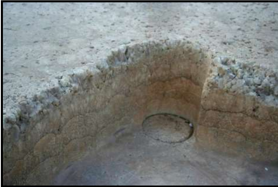
Evidence of core drilling in the hotep
