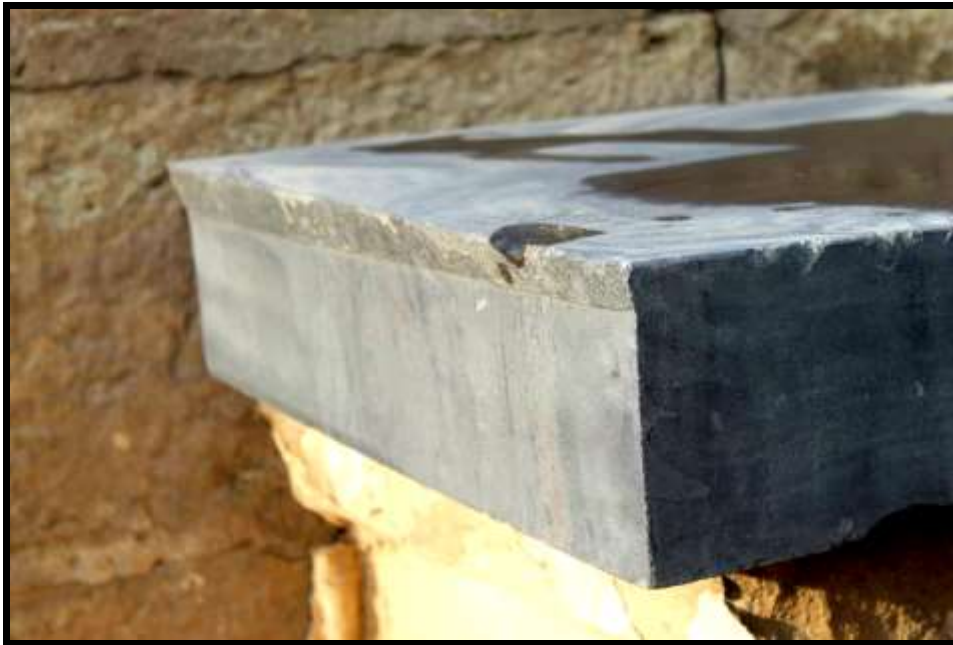
Obvious saw marks and termination of a cut
