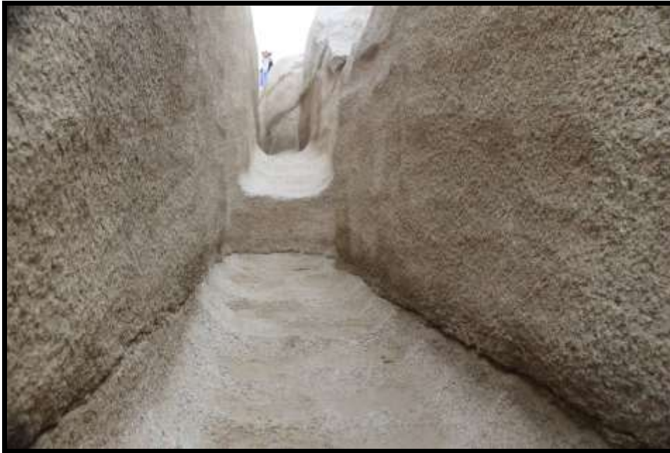
Trench at the unfinished obelisk showing crack
