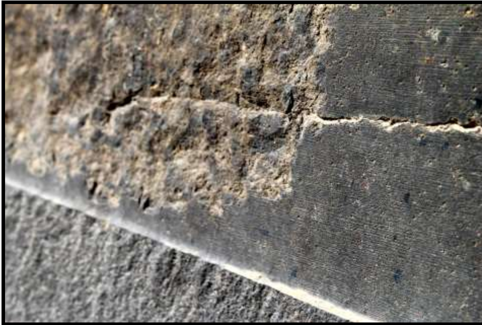
The saw was cutting at least 2 mm per revolution
