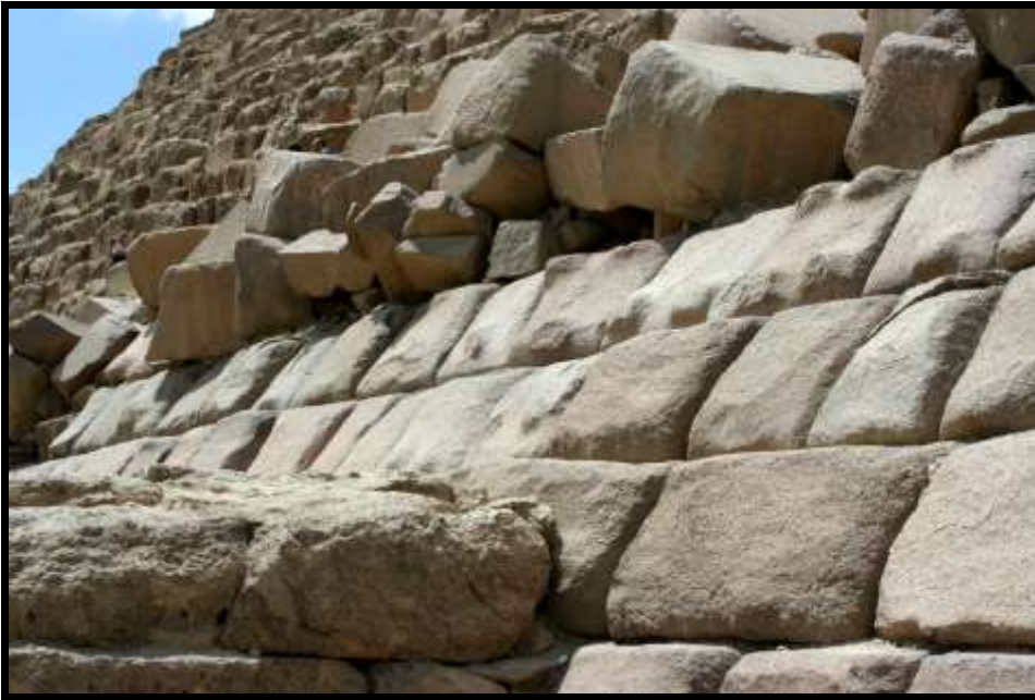
Detail view of the rose granite casing stones
