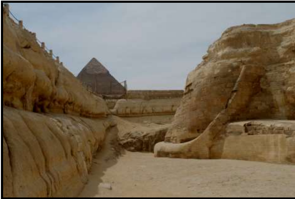
Weathering of Sphinx enclosure on the left of the photo
