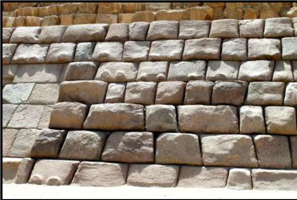
Casing stones on the Menkaure Pyramid with protrusions
