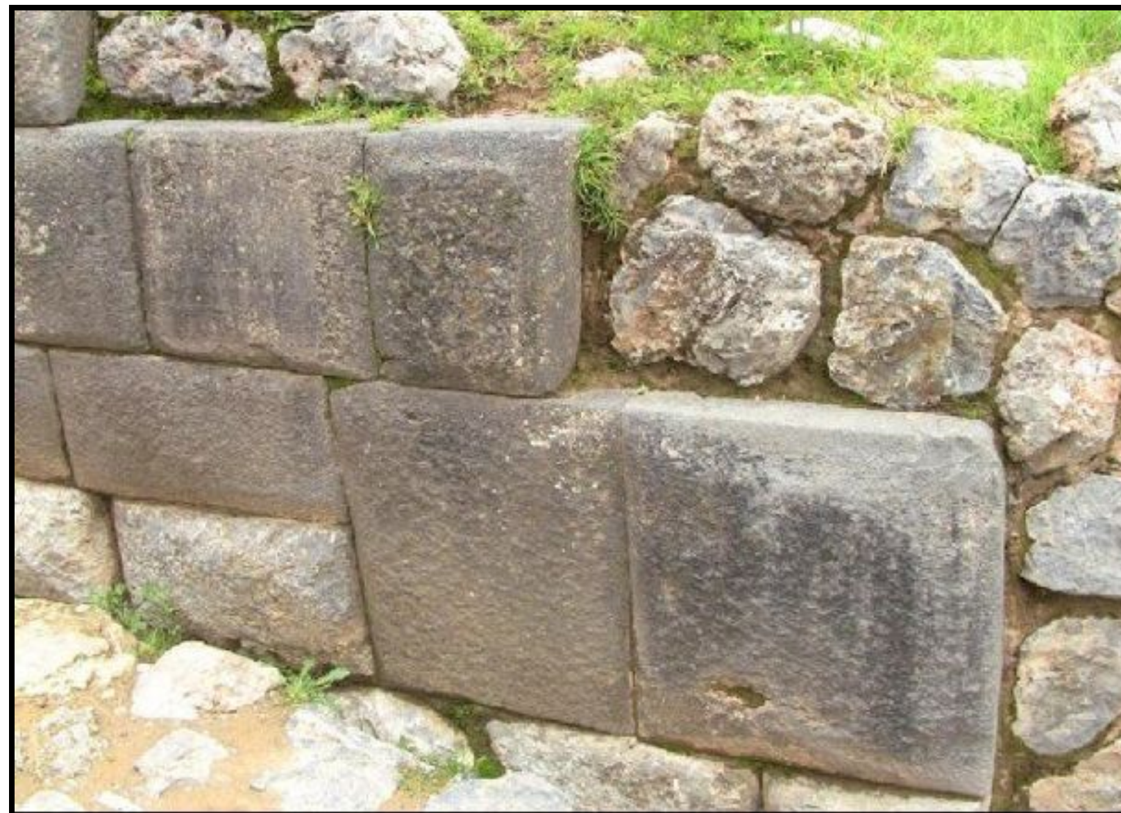
Part of the stone wall of the “circle” area showing two different construction styles
